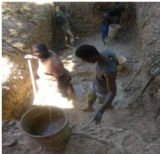
Digging new septic after Hurricane Laura
